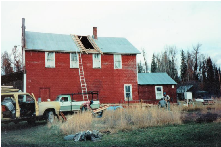
Replacing fire-damaged roof section at the Merc (top); Destroyed gasoline pumps (bottom)
