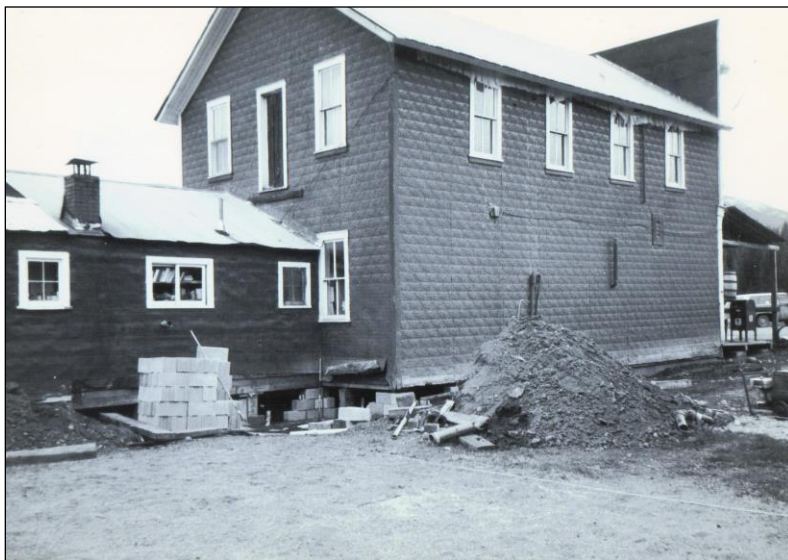
Putting a new foundation under the Mercantile in 1982 also involved removing the apartment on the south side of the building.
