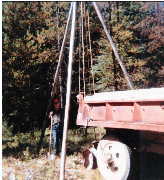
Ted Ross's apparatus for drilling water wells. He sank wells, on request, for families that purchased lots in the Skyline Acreage subdivisions.
