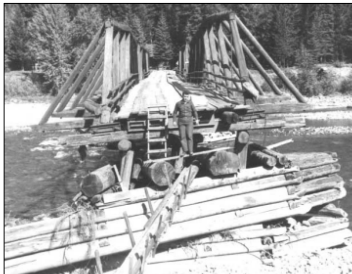
1964 flood damage to the pole bridge over the North Fork River.
